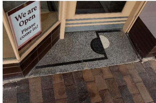
Terrazzo re-entrant floor to Shop 1
