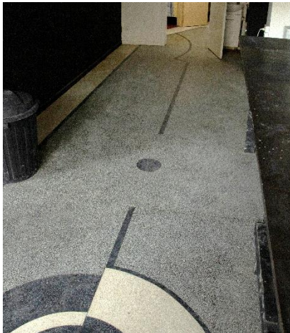
Side exit terrazzo floor
