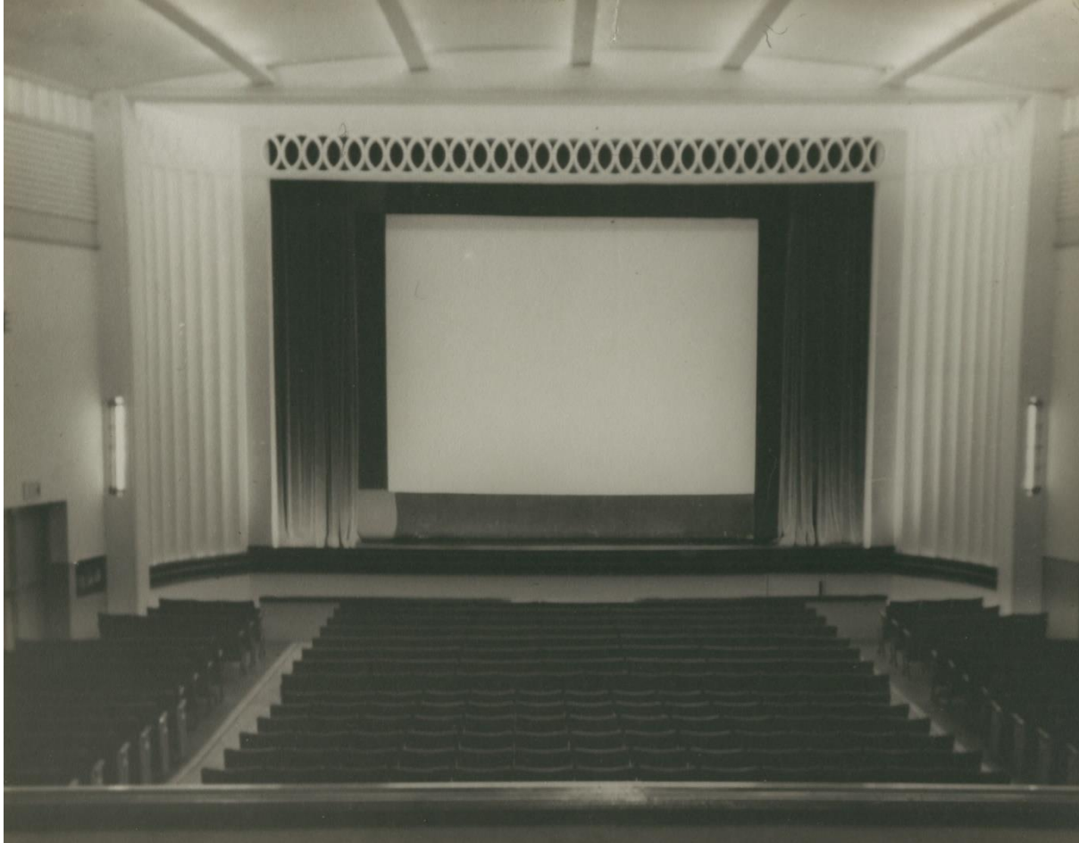
Victor Harbor Ozone Theatre auditorium before CinemaScope installation, 1955
