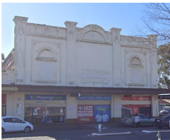
Former Alberton Ozone Theatre, 33 Fussell Place, Alberton (LHP)
