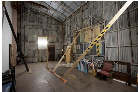
Interior stage house
