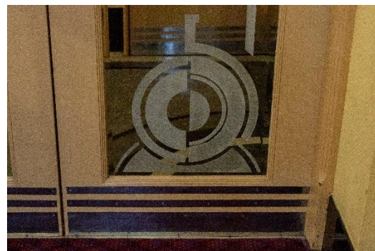
Details of doors between vestibule/ foyer, note sandblasted motif and chromed kickplates
