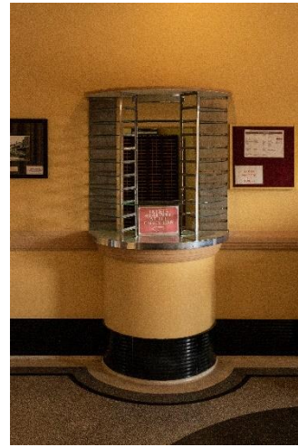
Ticket Box in vestibule, note curved black vitrolite skirting
