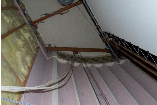
Original proscenium hidden behind screen with perforated fibrous plaster frieze at top
