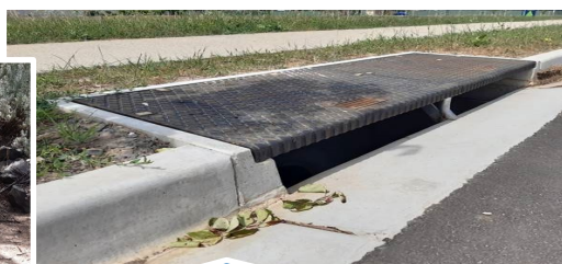
Stormwater Pits
