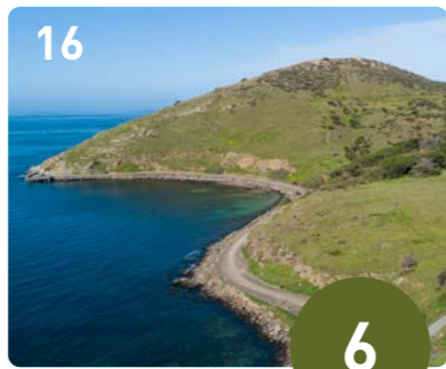
Upgrades to Franklin Parade (also known as Bluff Jetty Road)
