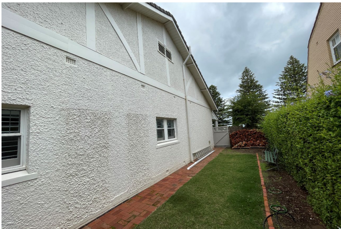
11 Bridge Terrace, Victor Harbor south western façade, where the infill of two original doors off bedrooms can be seen (GGA, 2023)
