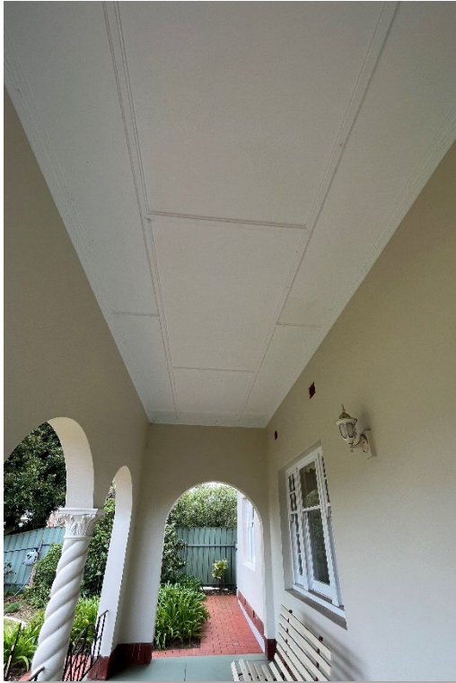
'Arcaded loggia' fibrous plaster and batten style soffit lining and painted concrete floor finish. (GGA, 2023)
