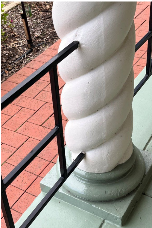
'Arcaded loggia' iron balustrade connection with column detail and entry glazed double door threshold. (GGA, 2023)
