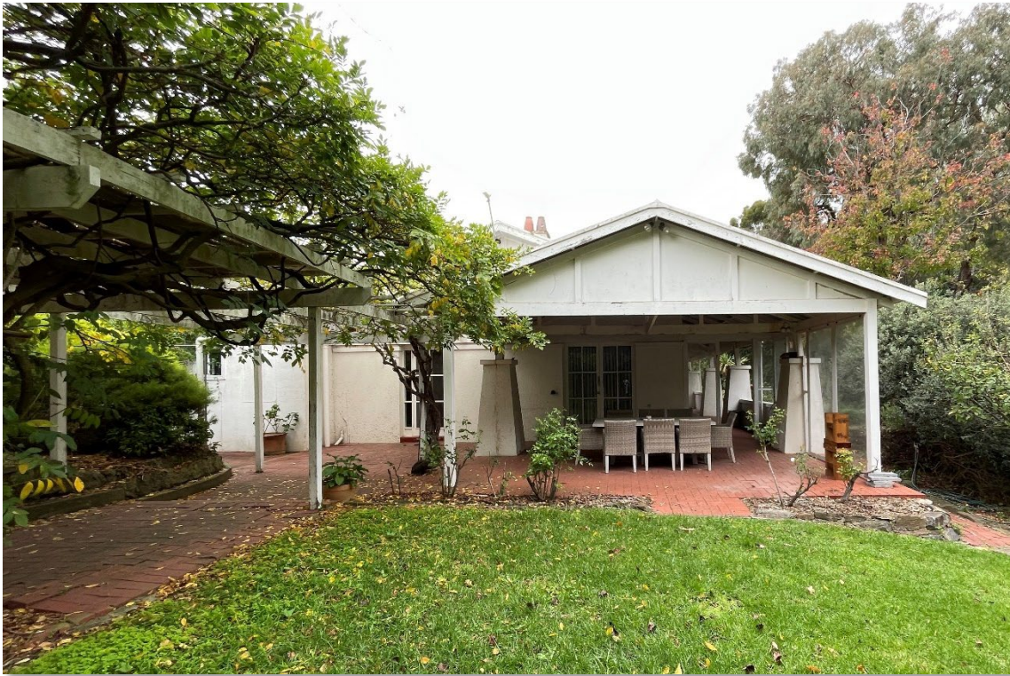
North western façade, showing non-original protruding gable addition to original gable and glazed double hinge double doors providing access to the verandah for all rooms. (GGA, 2023)
