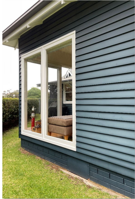
1 Bridge Terrace, Victor Harbor later sections of dwelling are constructed on concrete slab or brick plinths (GGA, 2023)
