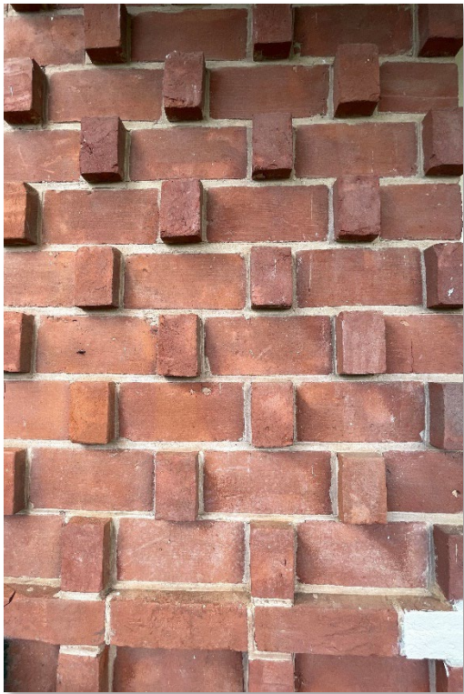
Unit 2, 27 William Street projecting 'Flemish' bond coursework and side of dwelling (GGA, 2023).
