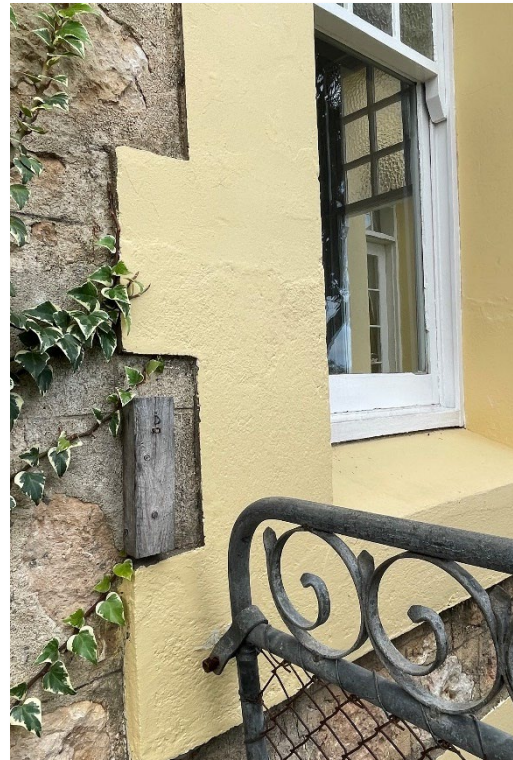
15 O'Leary Street, Victor Harbor original pier to side entry concealed below later timber deck and evidence of altered window through difference in texture of window reveal (GGA, 2023)
