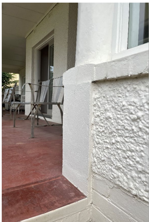
11 Bridge Terrace, Victor Harbor opening made to balustrade and lightweight infill with glazed brick step up to verandah (GGA, 2023)
