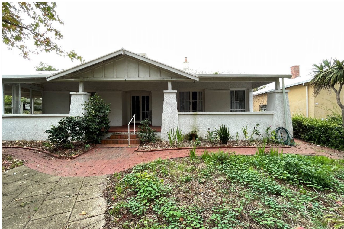
South western façade, showing protruding gable, centralised on the original verandah, 'lace' finish style stucco tapered piers, with matching balustrade infill and glazed double hinge double doors providing access to the verandah for all rooms. (GGA, 2023)
