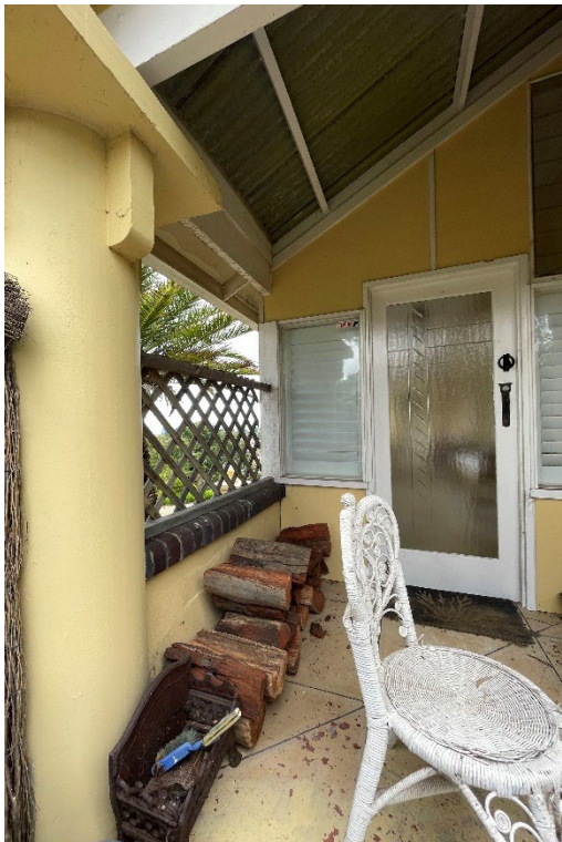
15 O'Leary Street, Victor Harbor infill to front verandah, with evidence of previous roofing material evident to the underside of the soffit and gable end façade detail (GGA, 2023)
