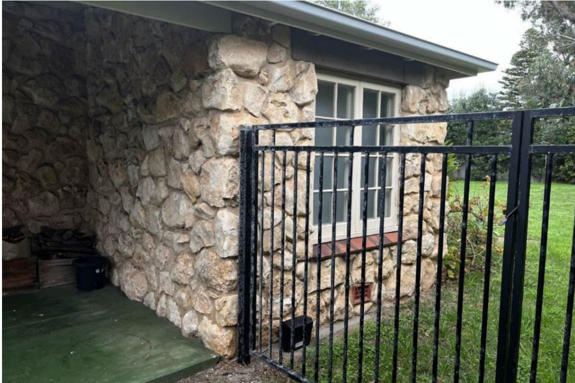
Rock face, randomised stone construction finish, with concrete render lintels and terracotta glazed style tile finish to sills (GGA, 2023)
