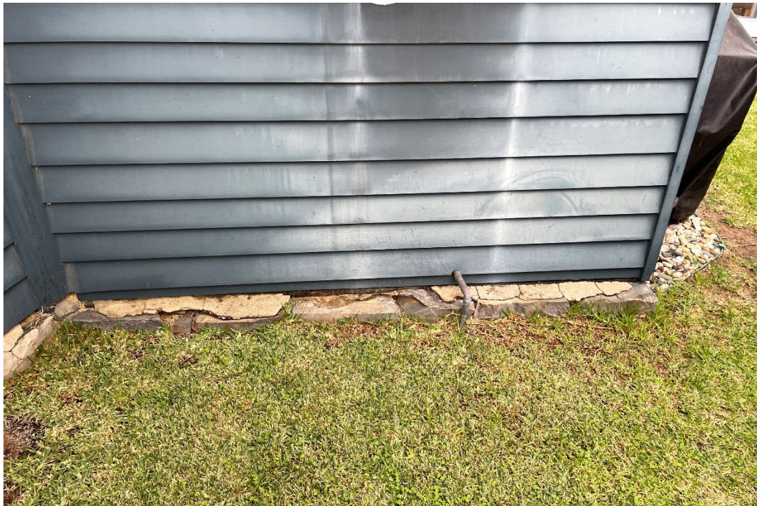
1 Bridge Terrace, Victor Harbor bluestone footings to what is likely an original section of dwelling (GGA, 2023)
