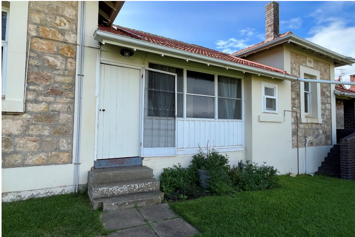
35-37 Seaview Road, Victor Harbor rear façade infill between hipped roof projections (GGA, 2023).
