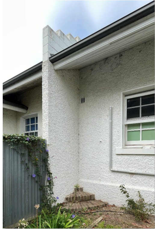
Photos taken to the rear, showing an infilled door opening at the location of the new dividing wall. (GGA, 2023)
