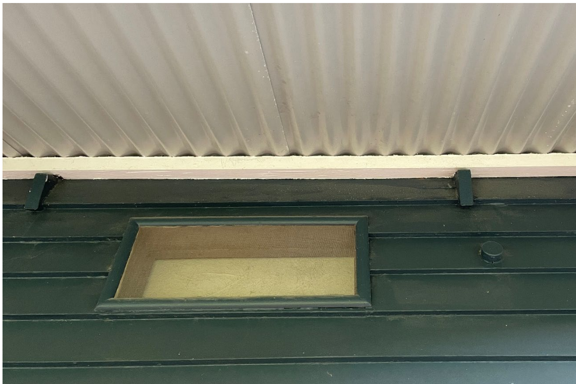
1 Bridge Terrace, Victor Harbor original section of dwelling where eastern section of building has been removed and rafter appear to have been cut (GGA, 2023)
