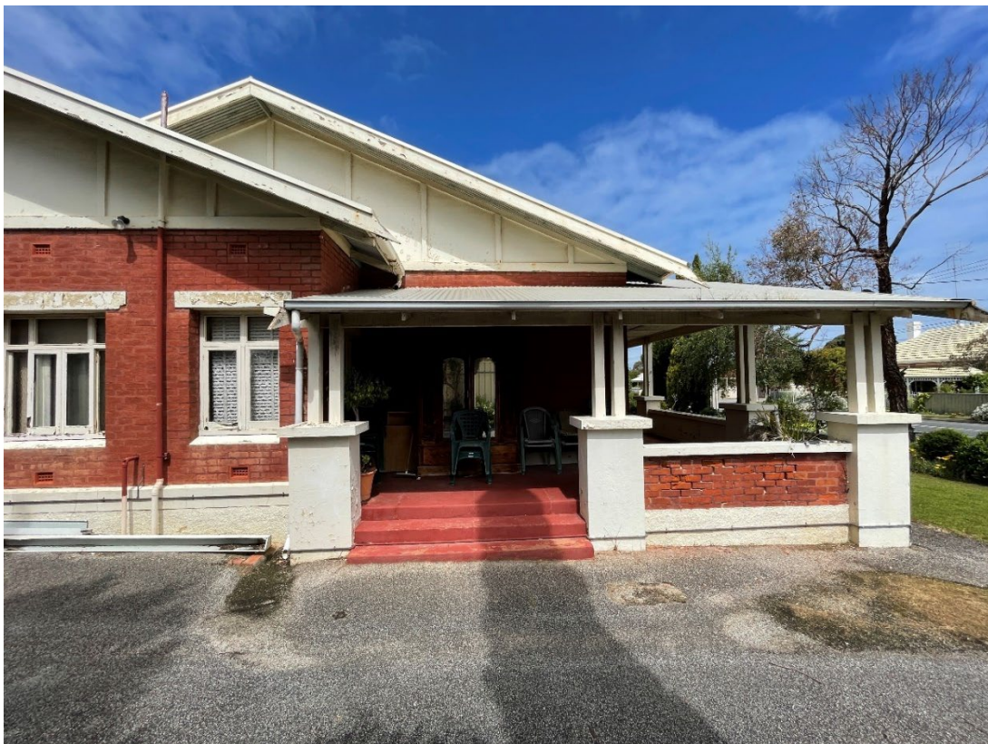
Verandah detail showing paired timber columns on rendered bases, brick infill to verandah wall (GGA, 2022)
