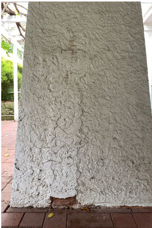
North western façade verandah pier, showing evidence of original masonry balustrade between piers having been removed to this façade. (GGA, 2023)
