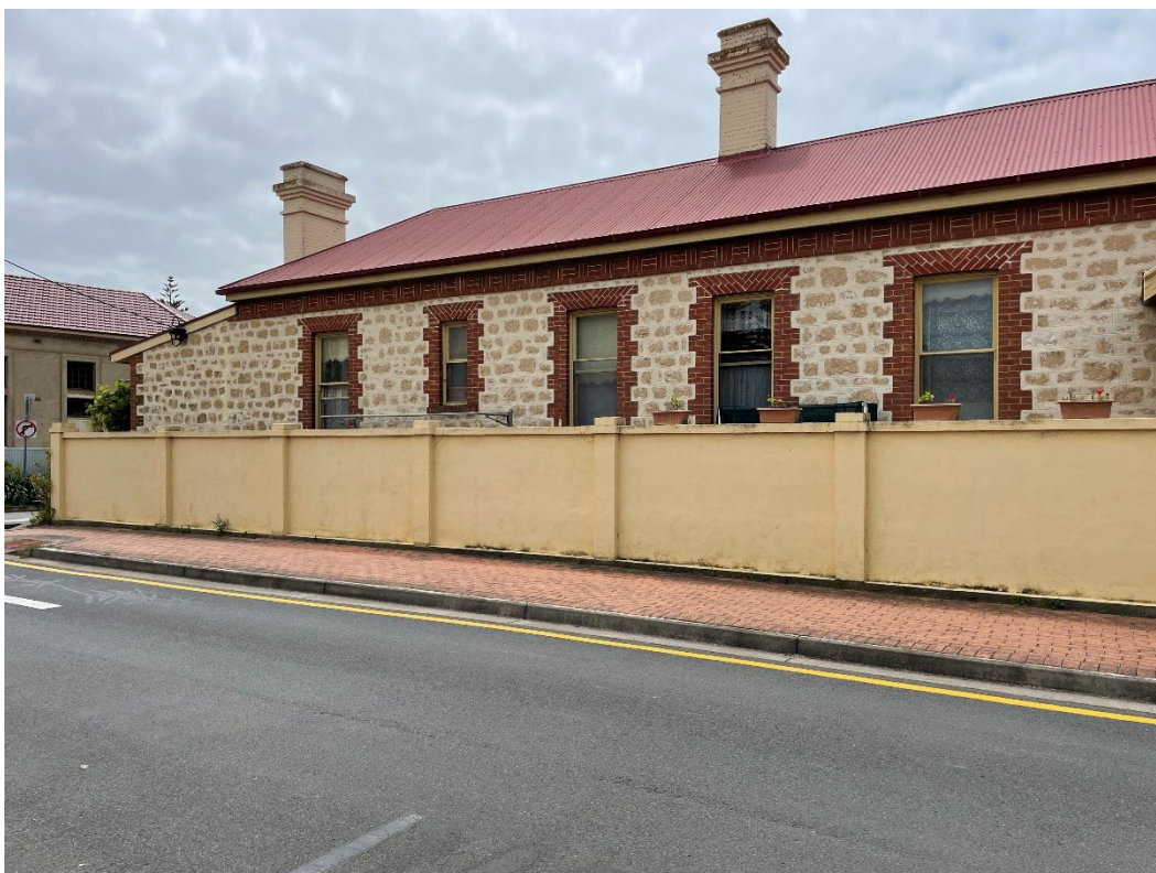
Side wall showing red brick window dressings and painted chimneys; later fence (GGA, 2023)
