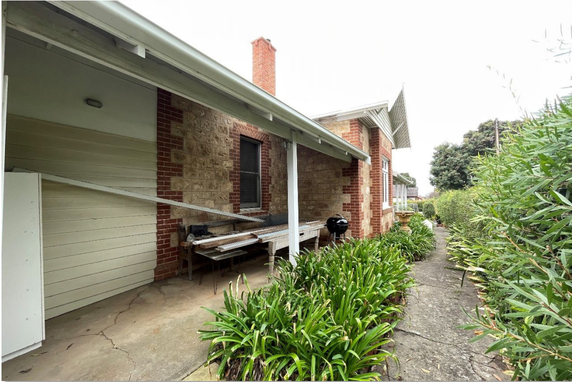
Western side of front façade, showing protruding gable form, extension of main roof past external walls to form verandah and brick chimney. (GGA, 2023)
