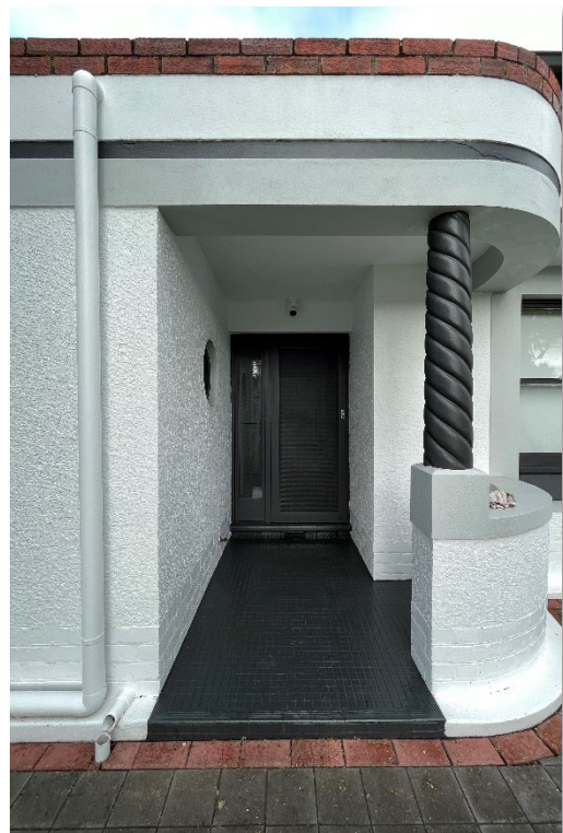
19 Hill Street, Victor Harbor entry portico detailing and small mosaic tile floor finish (with later paint finish) (GGA, 2023)
