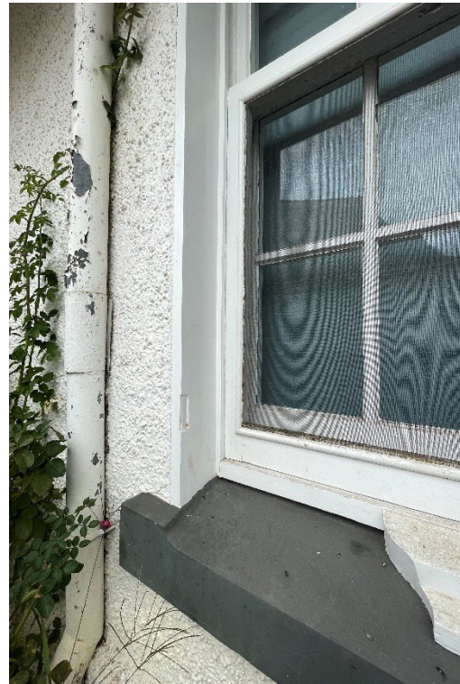
Evidence remains, indicating shutters were originally installed to the windows. (GGA, 2023)
