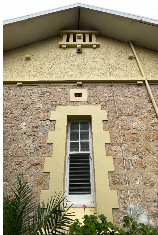
15 O'Leary Street, Victor Harbor infill to front verandah, with evidence of previous roofing material evident to the underside of the soffit and gable end façade detail (GGA, 2023)
