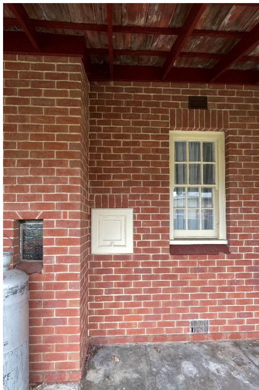
12-16 Burke Street, Victor Harbor – what is thought to be a milk delivery hatch to the right of the kitchen fireplace and the underside of the verandah (GGA, 2023)
