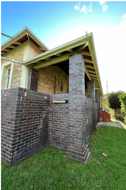
35-37 Seaview Road, Victor Harbor rear eastern verandah and soffits exposed to underside of roof finish (GGA, 2023).
