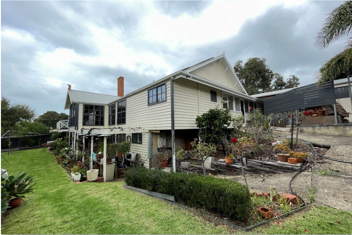
Non-original rear addition, infill and reconstruction of verandah (owner noted rear original rear verandah was replaced, within original footprint, due to structural concerns). (GGA, 2023)
