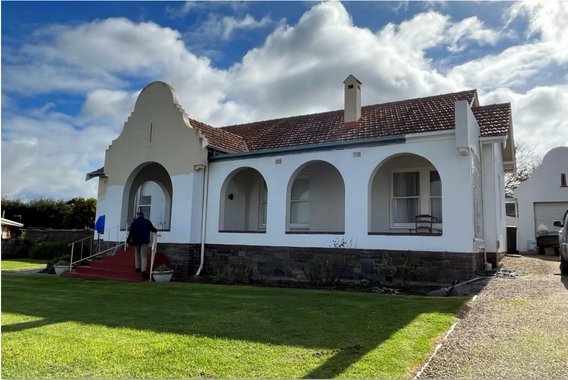
Front façade, showing 'arcaded loggia', decorative parapet, roofing tiles, chimney, concrete stairs plinth. (GGA, 2023)
