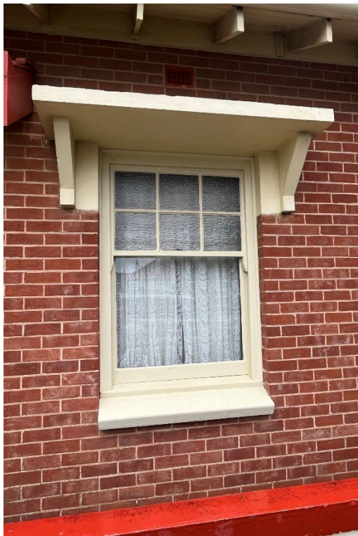
Window detail, along Lindsay Street, with concrete awning over (GGA, 2023)
