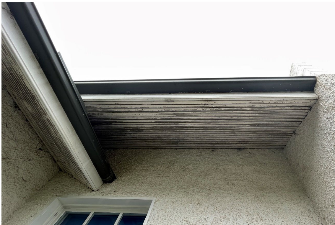
Thin timber batten linings remain to the eaves at the rear of 32 Esplanade. (GGA, 2023)
