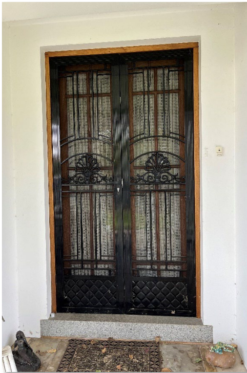
Glazed double entry doors behind non-original security screen doors and terrazzo finish sill (GGA, 2023)
