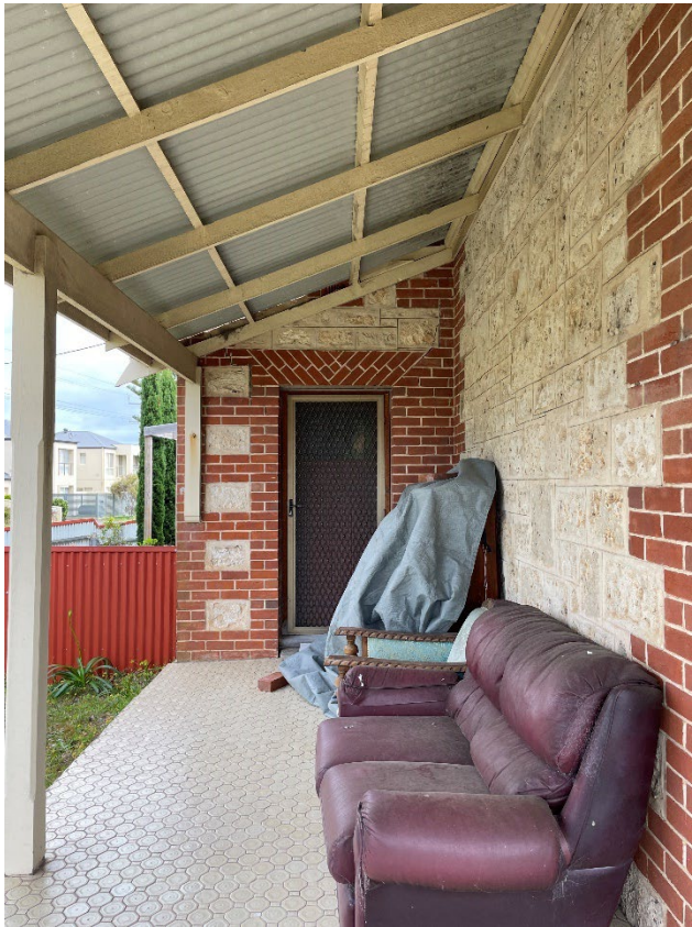
39 George Street, porch showing later tiles, limestone face stonework, brick quoins and dressings (GGA, 2022)
