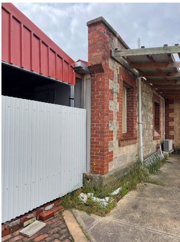
39 George Street, parapet to rear section with later metal clad additions (GGA, 2022)
