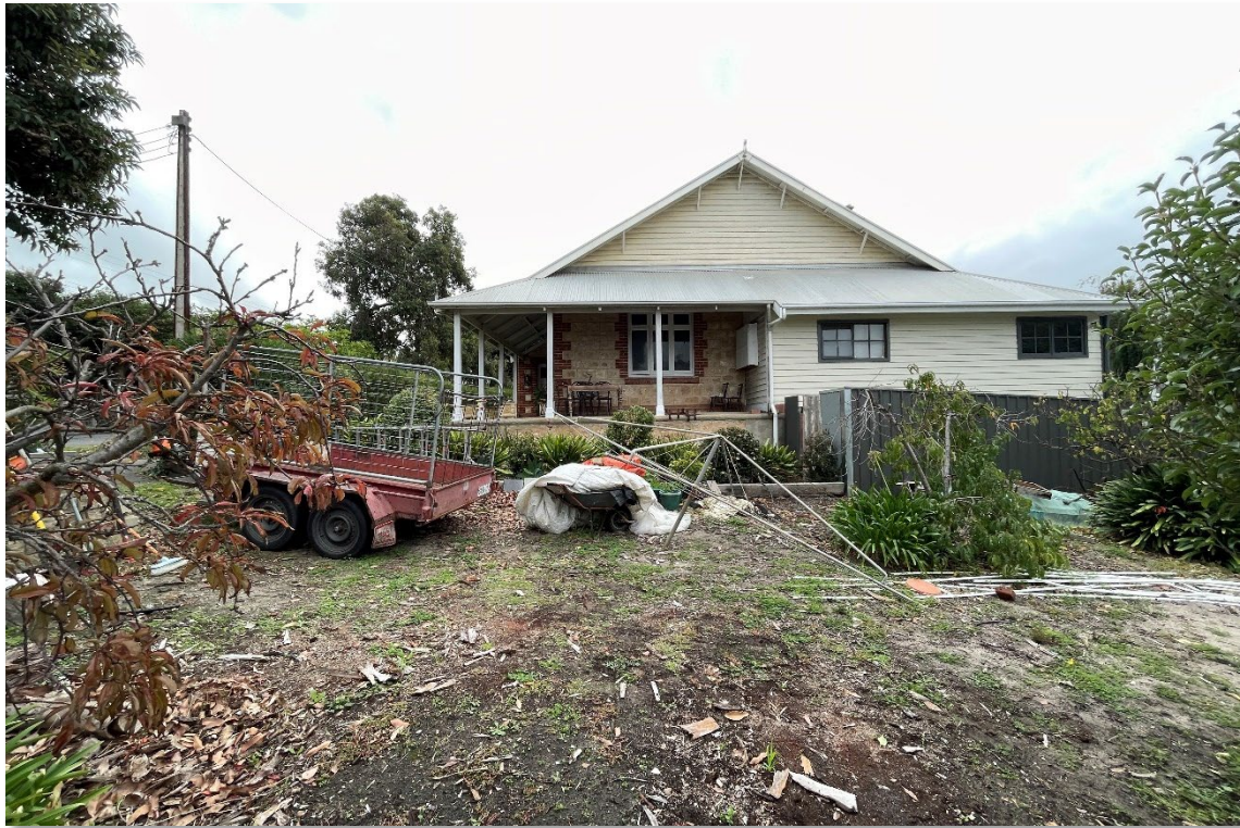
South eastern main roof gable end, showing weatherboard gable end finish, timber bracket and scroll detailing. (GGA, 2023)
