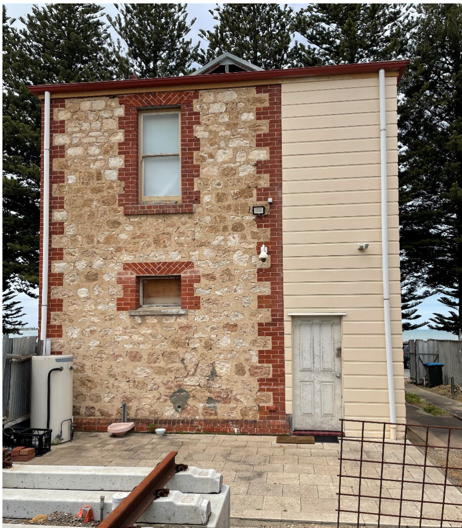
Rear elevation showing later lightweight infill to right hand side of image (GGA 2022)
