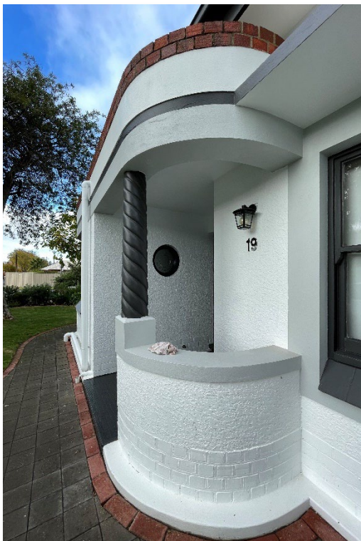
19 Hill Street, Victor Harbor entry portico detailing and small mosaic tile floor finish (with later paint finish) (GGA, 2023)
