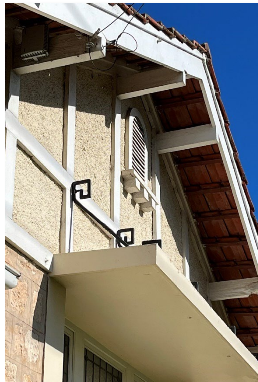
35-37 Seaview Road, Victor Harbor rear eastern verandah and soffits exposed to underside of roof finish (GGA, 2023).
