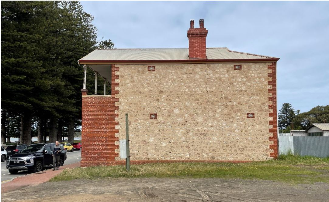
Side wall view showing face limestone work, brick detailing, brick chimneys (GGA 2022)
