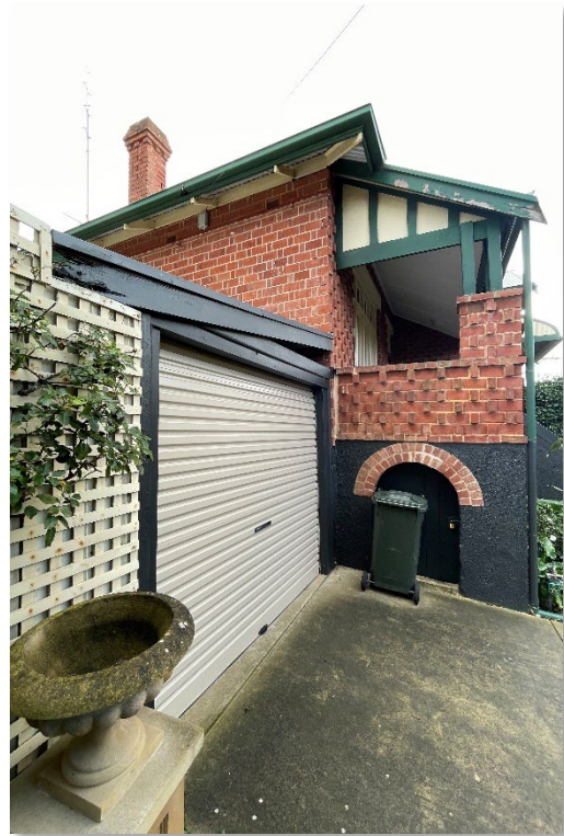
Unit 2, 27 William Street projecting 'Flemish' bond coursework and side of dwelling (GGA, 2023).
