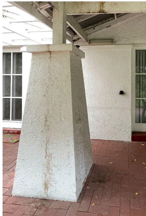
North western façade verandah pier, showing evidence of original masonry balustrade between piers having been removed to this façade. (GGA, 2023)
