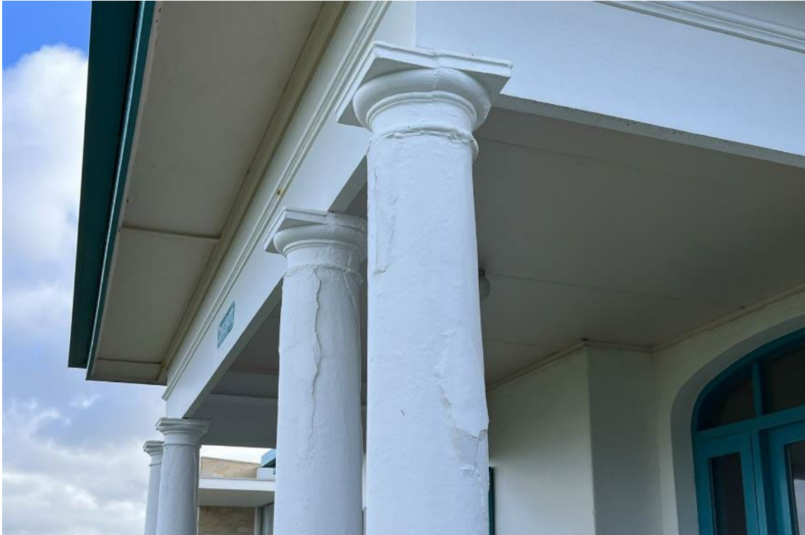
Concrete, doric style, columns to 'loggia', showing signs of 'concrete cancer' (GGA, 2023)
