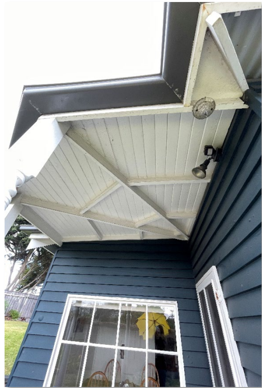
1 Bridge Terrace, Victor Harbor original section of dwelling timber rafters are finished with a curve, possibly indicating that the roofing finish was eyelash in profile and underside of porch (GGA, 2023)
