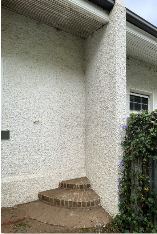
Photos taken to the rear, showing an infilled door opening at the location of the new dividing wall. (GGA, 2023)
