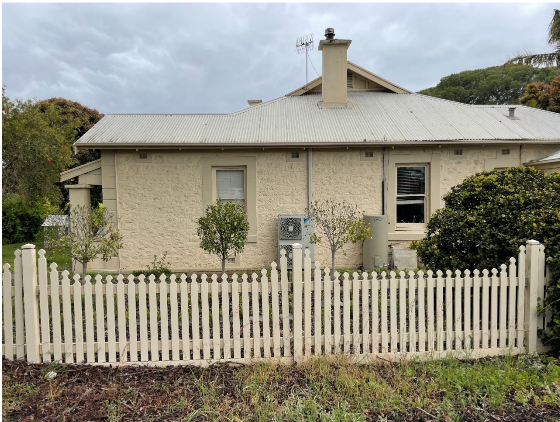
Side elevation showing painted stonework, rendered chimney and timber detail to roof gable (GGA 2022)
