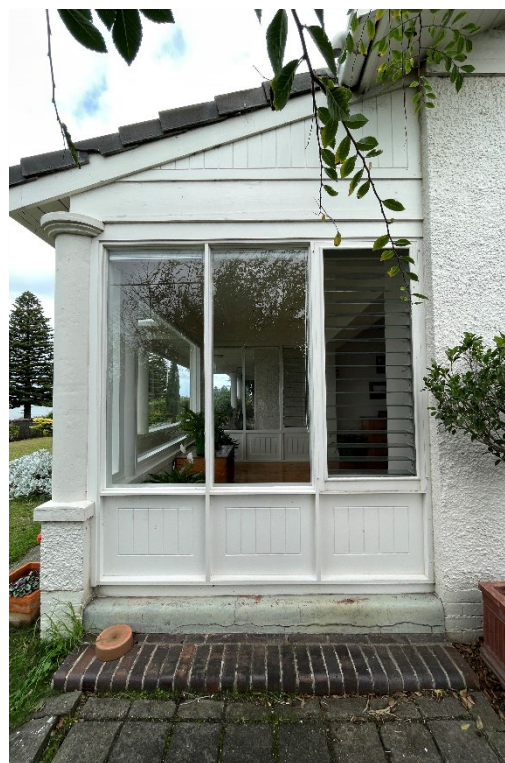
11 Bridge Terrace, Victor Harbor opening made to balustrade and lightweight infill with glazed brick step up to verandah (GGA, 2023)
