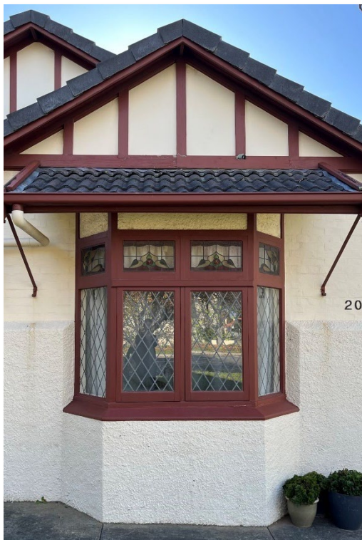
Bay window to the front façade protruding portico and entry archway to the porch under the catslide style roof. (GGA, 2023)
