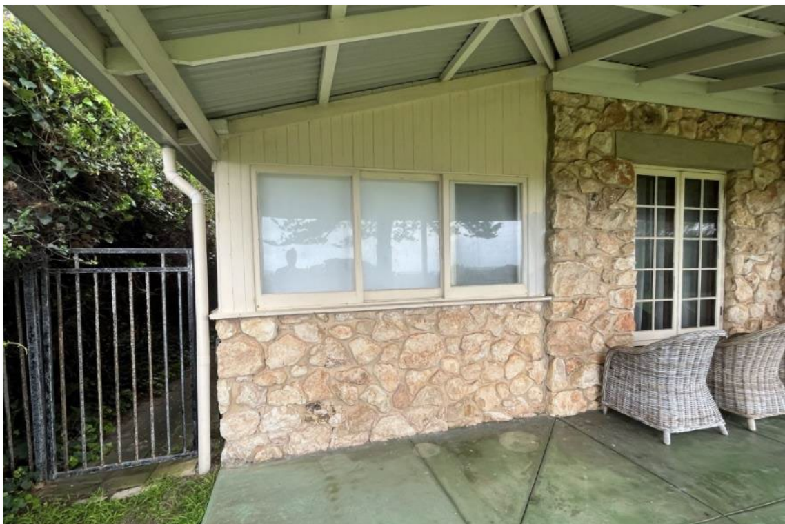
Later infill addition to side façade, under extension of roof as verandah (GGA, 2023)
