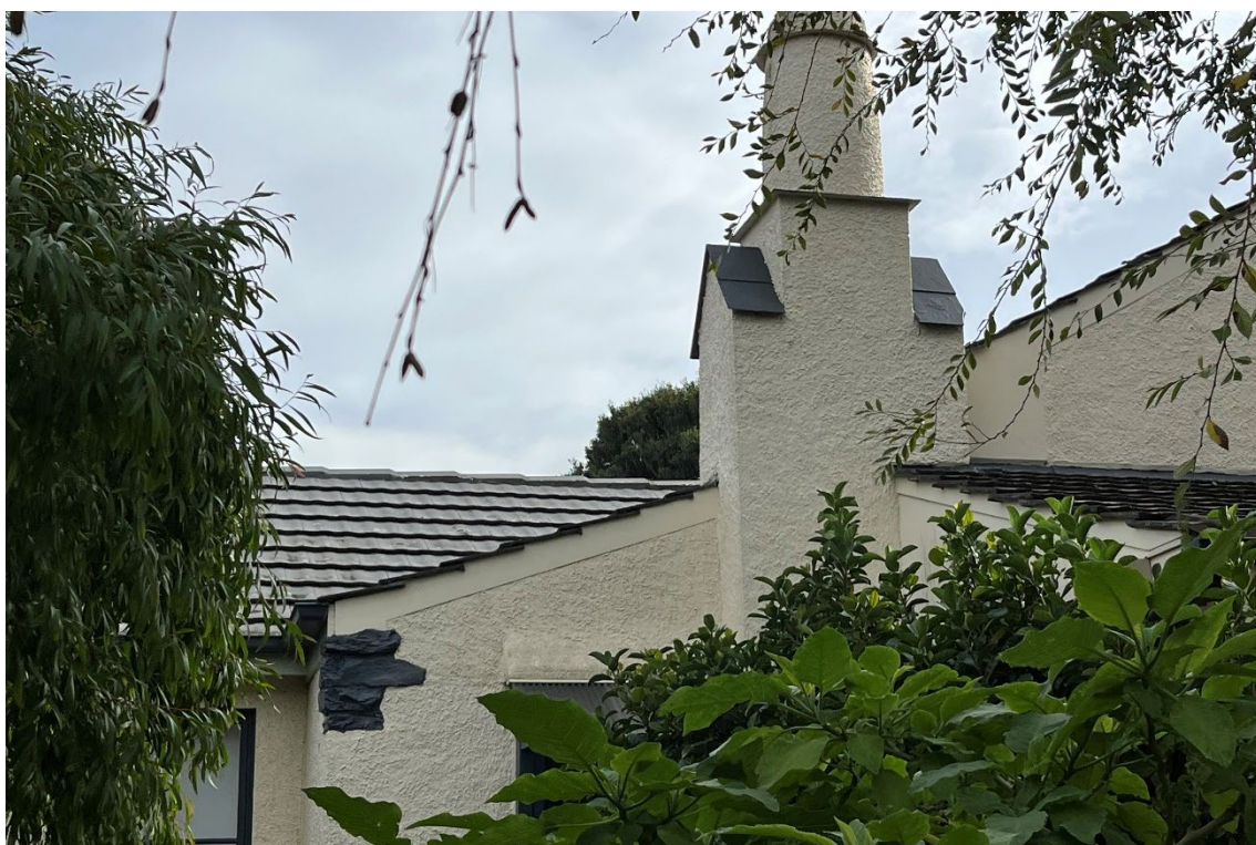
19 -21 Grantley Avenue, Victor Harbor chimney example and bluestone (later paint finish) coursing detail at gable pitching point (GGA, 2023).
