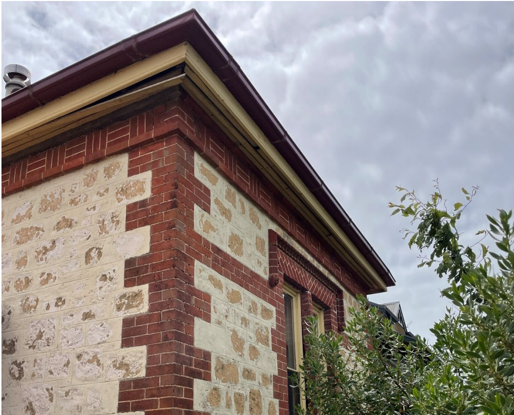
Limestone walling, brick quoins and decorative brick string course under eaves (GGA, 2023)
