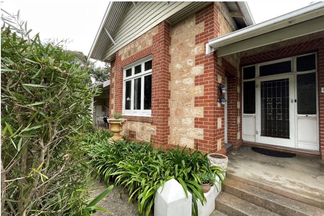
Western protruding gable form showing timber birdboard soffit lining and weatherboard gable end finish. (GGA, 2023)
