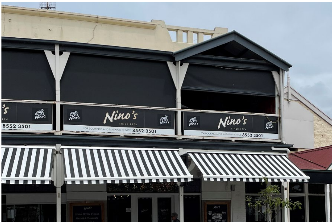
Verandah detail with timber brackets and end gable detail, masonry parapet behind (GGA 2022)
