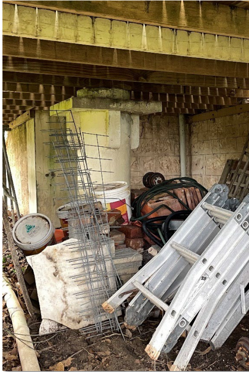
15 O'Leary Street, Victor Harbor original pier to side entry concealed below later timber deck and evidence of altered window through difference in texture of window reveal (GGA, 2023)
