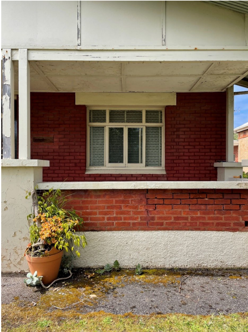
Verandah detail showing rendered and brick plinth, multi-pane timber windows with rendered lintel beyond (GGA, 2022)
