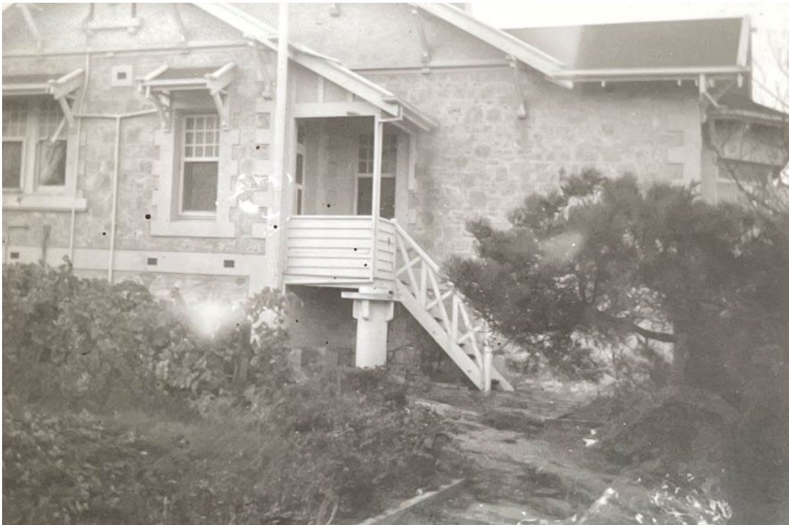
Photograph taken from the south west, looking at the southern corner of the dwelling. Items of note include the altered stair, entry landing and gable extension, sash window and door, roof finish, protective window awnings, and timber bracket details to gable ends. Owner supplied image, year unknown.
