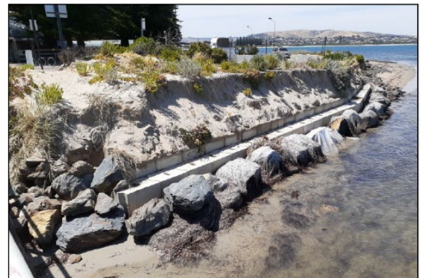
March 2017 and November 2019 A gentle slope from car park level down to the beach was severely eroded all the way along between the causeway and the boat ramp. A block wall, topped with a sand dump and revegetation was built.
