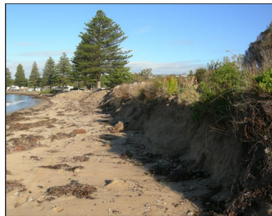
June 2012 Opposite house numbers 69 to 71. Severe erosion
