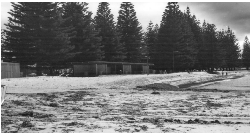
Figure 19. Sand nourishment of 3000m 3 in March 1976 because sand levels were dropping on the beach and the seawall undermined and damaged (Scan: CPB, 19760301).
