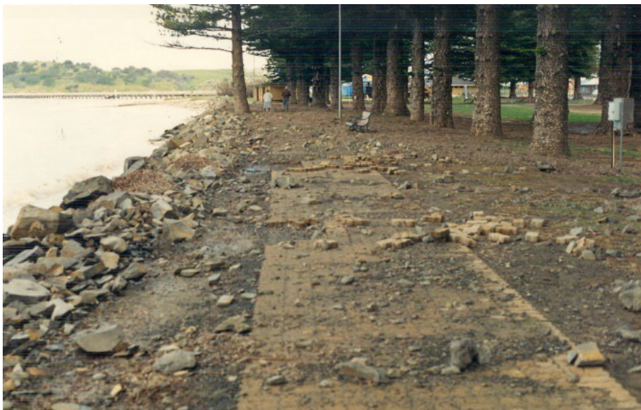
Figure 22. Debris from storm event 1989. Council reports that seaweed debris is often deposited from moderate storm action in this location (Photograph CPB, 19890912).
