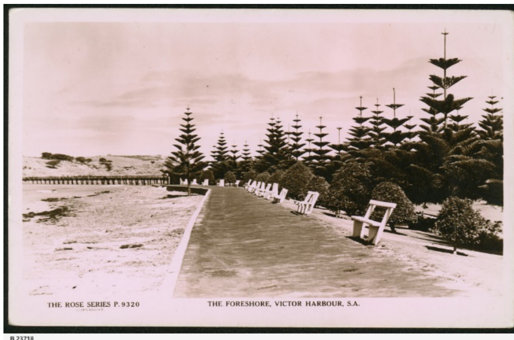
Figure 17. Seawall installed in 1920. The promenade area was likely raised with imported fill and the slope behind backfilled (SA State Library, 1937, B-23718).
