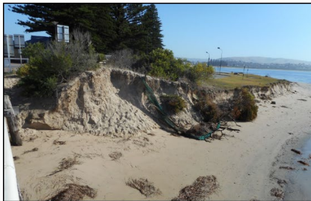
March 2017 and November 2019 A gentle slope from car park level down to the beach was severely eroded all the way along between the causeway and the boat ramp. A block wall, topped with a sand dump and revegetation was built.
