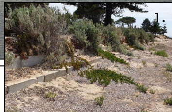
1. Concrete block seawall – installed 2015 as a trial.
