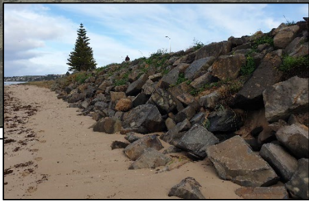
2. Rock revetment – well constructed and in sound condition
