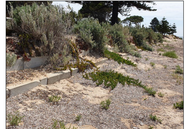
Figure b. Cement blocks 5 tiers high, in vicinity of Fell Street (Photograph – M. Western, 2021).
