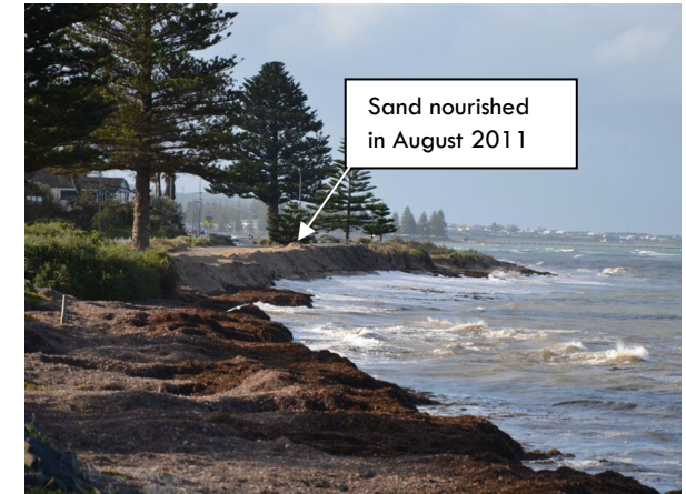
Figure e. Storm impact between Fell Street and Fountain Ave, 4 June 2012 (Photograph - Coast Protection Board, 20120604).
