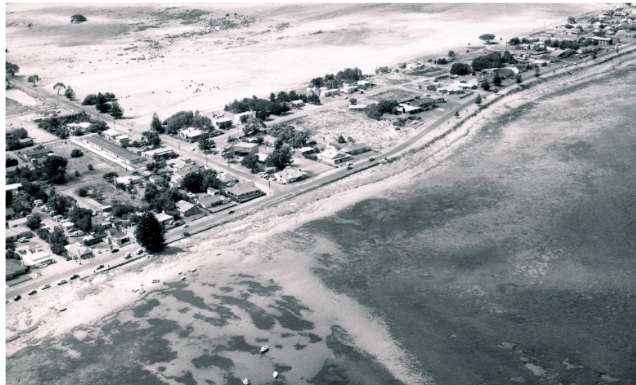
Figure a. The backshore in the vicinity of Yilki and Tabernacle Road was an unvegetated slope back to the road (which appears to have a seawall, most likely constructed in 1950s)
