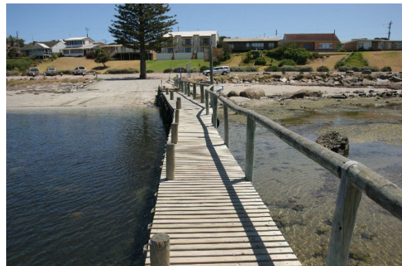
Figure c. Boat ramp constructed in 1987, jetty added in 1998 (Photograph – Coast Protection Board, 20061205)
