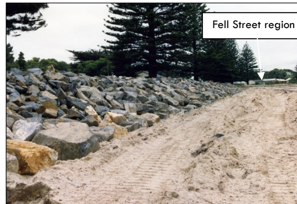
Figure a. Rock revetment extended Jan 2005 (after storms in 2004). (Photograph - Coast Protection Board, 20050101).
