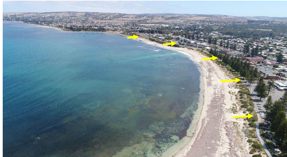
Figure a. The Esplanade Beach – erosion in the second half of this century is likely to impact carpark, reserve, visitor centre.
