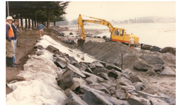
Figure c: Rock revetment installed (Photograph: CPB, 1 March 1987)
