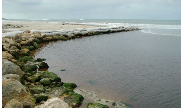
Figure a: Hindmarsh River – training groyne (CPB, 20040810).
