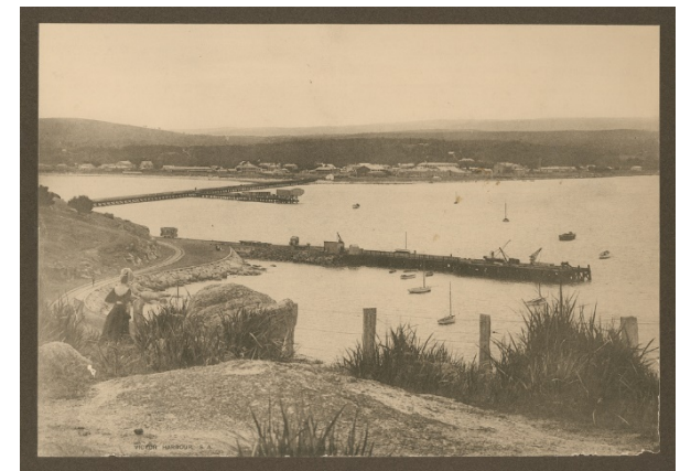
Figure a: Victor Harbor, 1910, causeway constructed to the island and 'working jetty' established (State Library of SA, B-17978).
