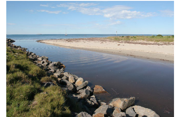
Figure c: Mouth of Inman River realigned, and rock training wall added in 1997. (CPB, 20070724).
