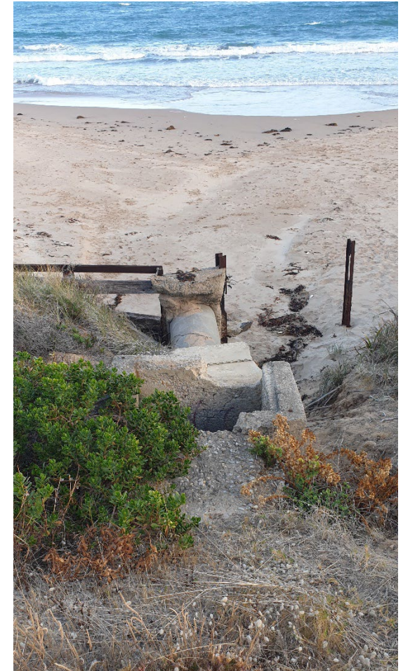
Figure b. The outlet (52) is in poor condition (not the focus of this assessment). Note the lower sand levels and seaweed strands which demonstrates that actions of the sea area interacting with this location.
