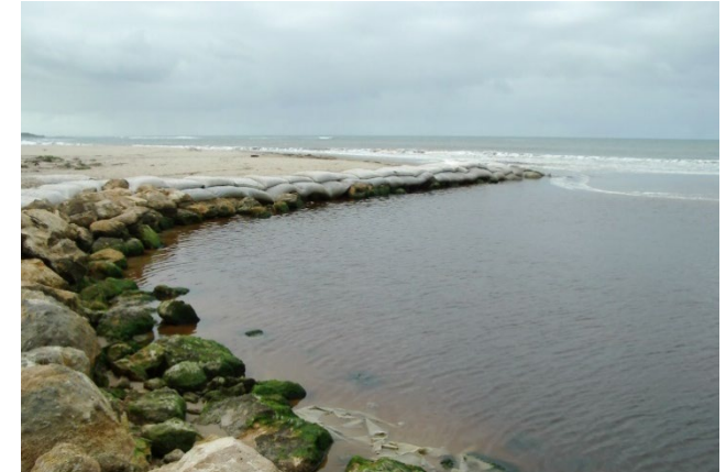
Figure d: Hindmarsh River outlet, 2004. Sandbags were added to the rock training wall. (Coast Protection Board).
