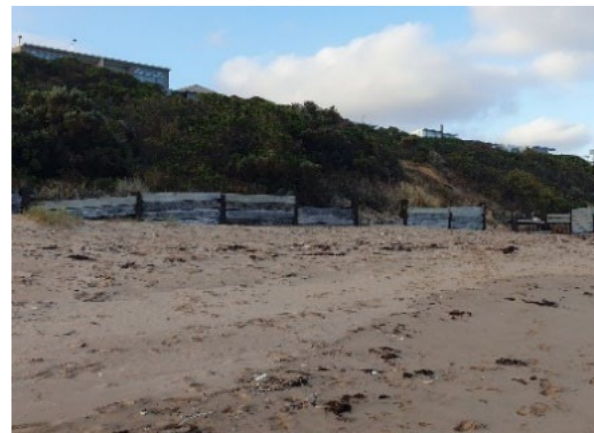
Figures c, d: The retaining wall is visible at two locations where storm water outlets have prevented the dunes from accreting.
