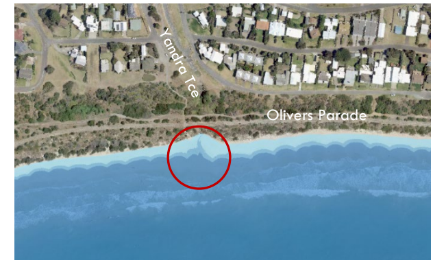
Figure b: Storm water outlet in the vicinity of Yandra Tce lowers sand levels on the beach.
