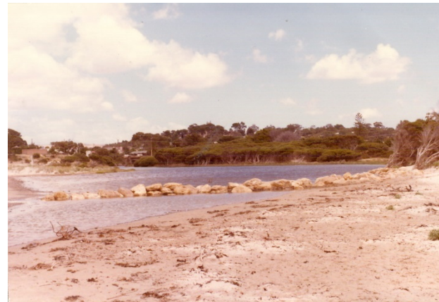
Figure c: Hindmarsh River outlet, 1984. Rock training installed (Coast Protection Board).
