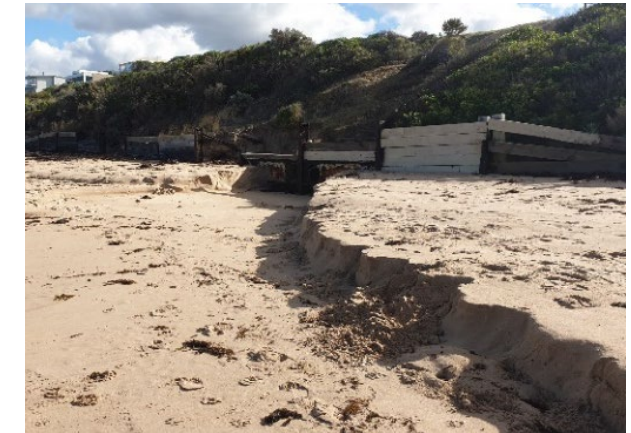
Figures c, d: The retaining wall is visible at two locations where storm water outlets have prevented the dunes from accreting.
