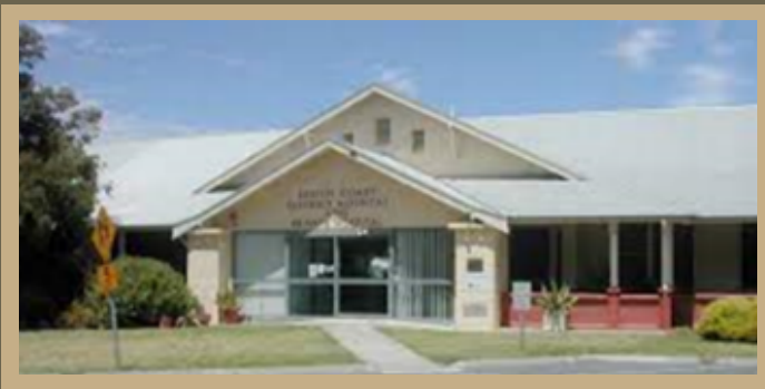
The South Coast District Hospital
