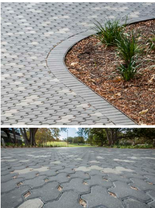
Permeable Pavers Eco trihex interlocking unit pavers (trafficable) Finish: Charcoal, honed finish Supplier: Adbri Masonry
